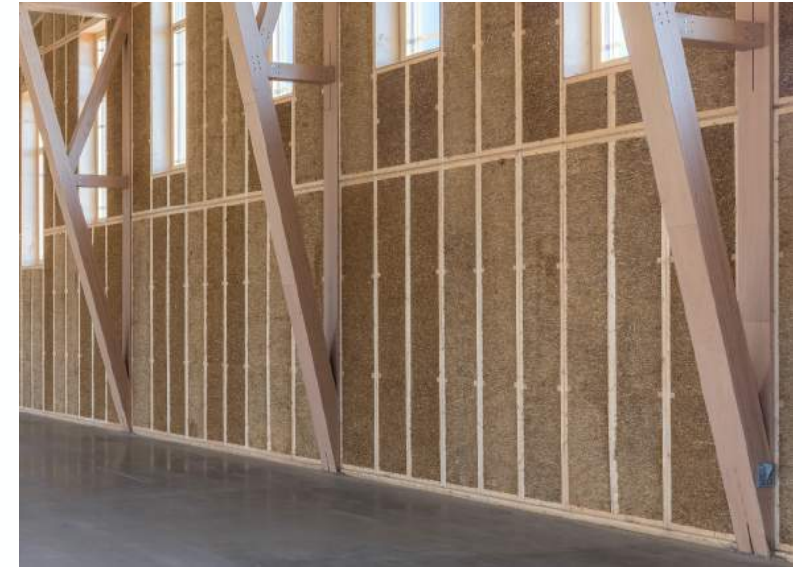
EcoCocon infill panels between timber frame.
