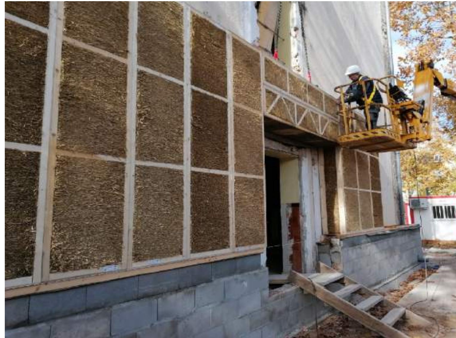
Self supporting structure (façade renovation).
