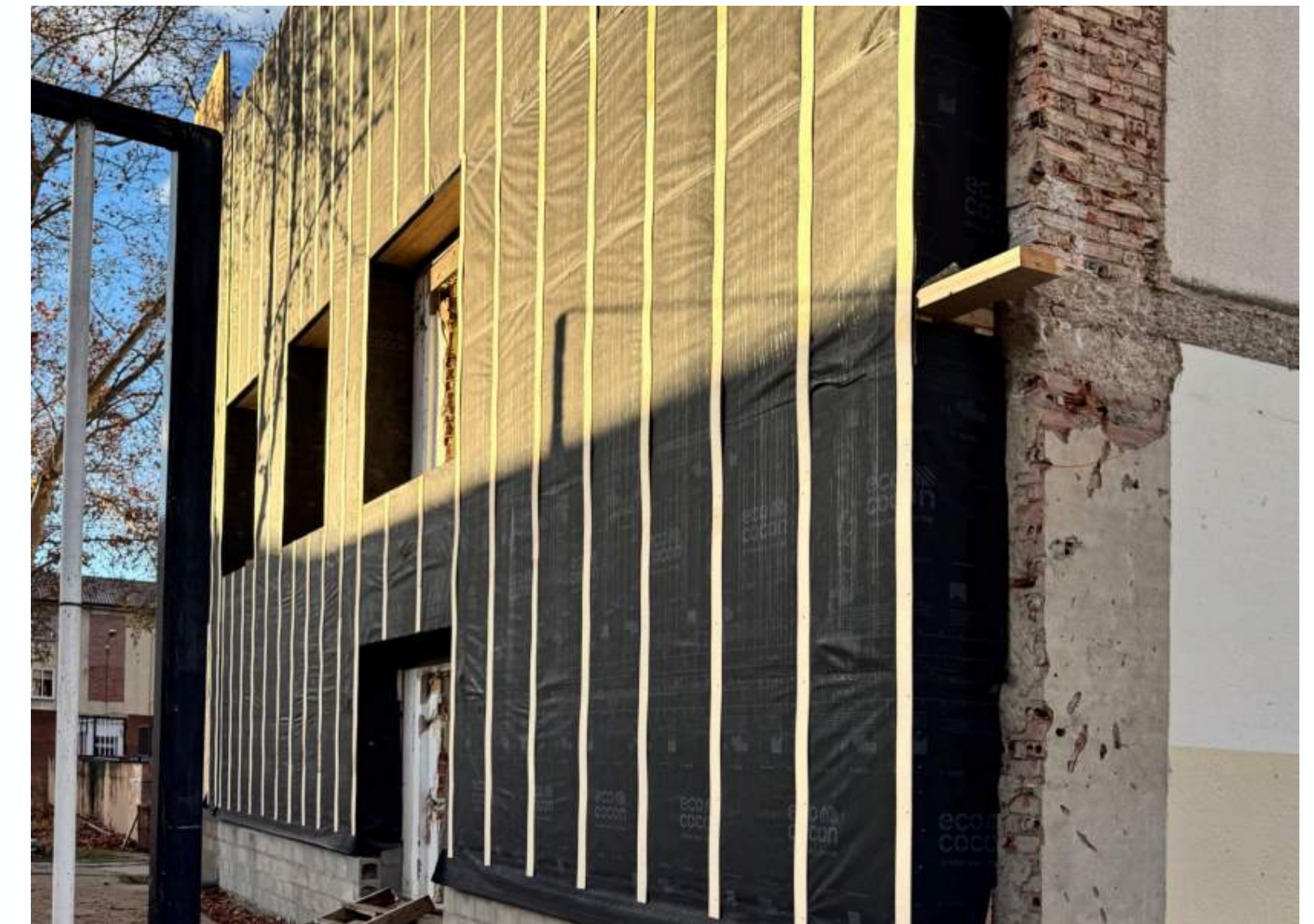
Self-supporting structure (façade renovation).
