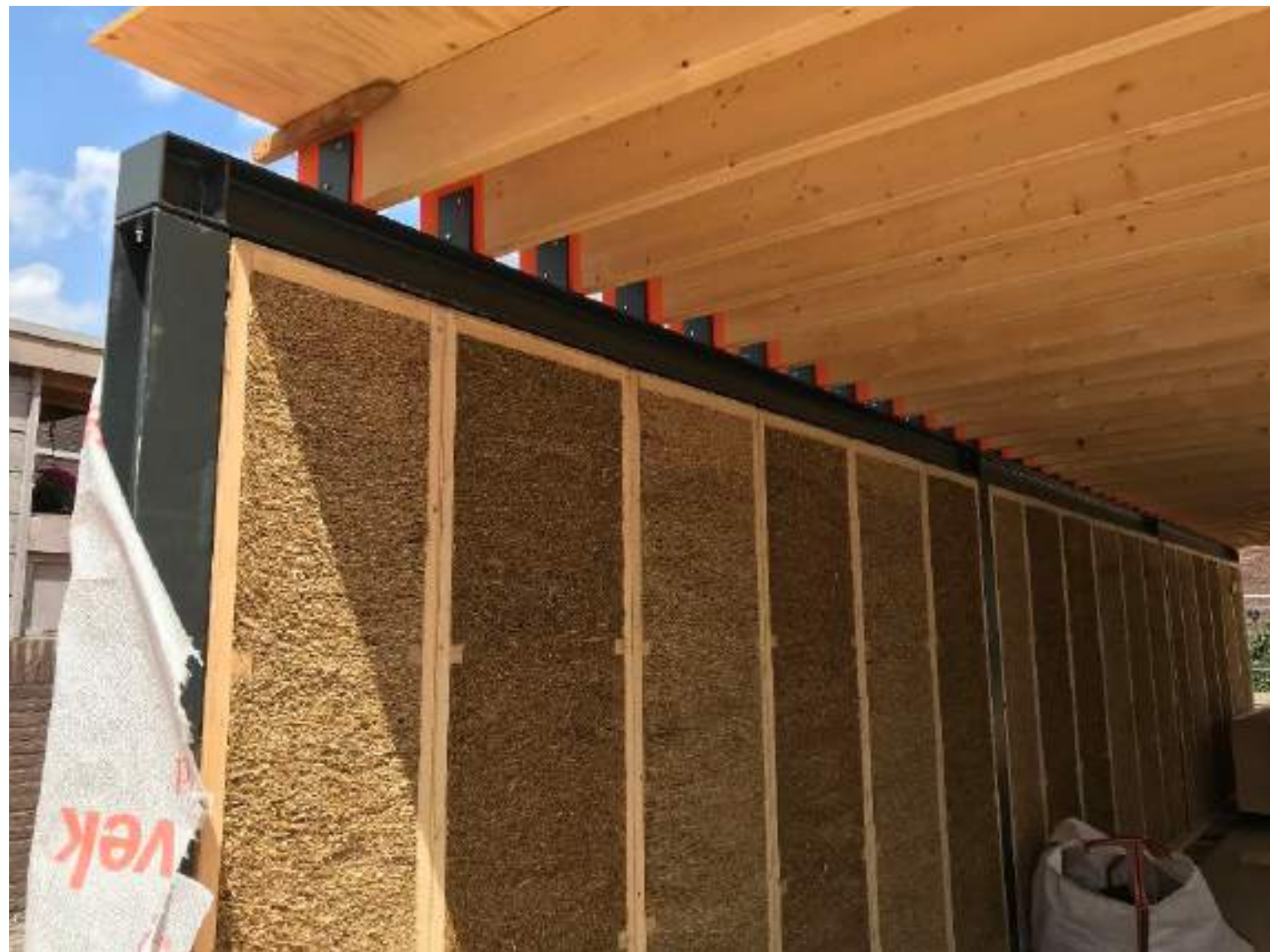
Non-load bearing walls (infill panels).
