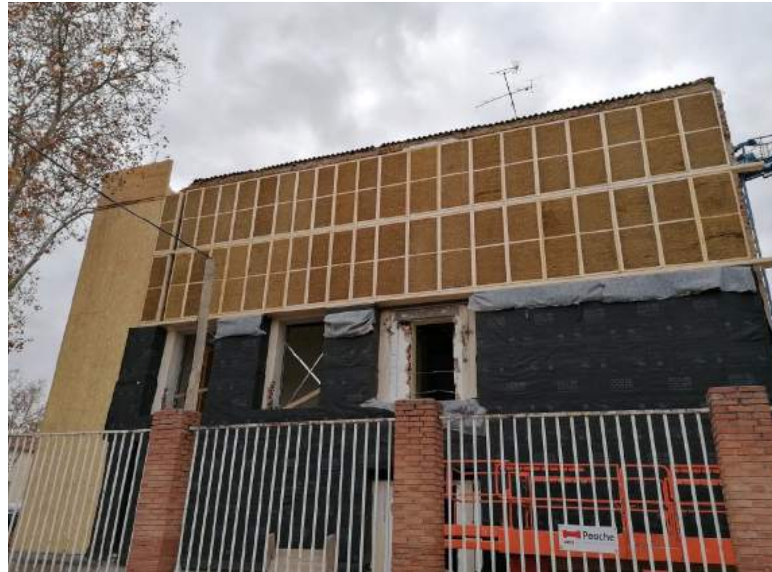
Self-supporting structure (façade renovation).
