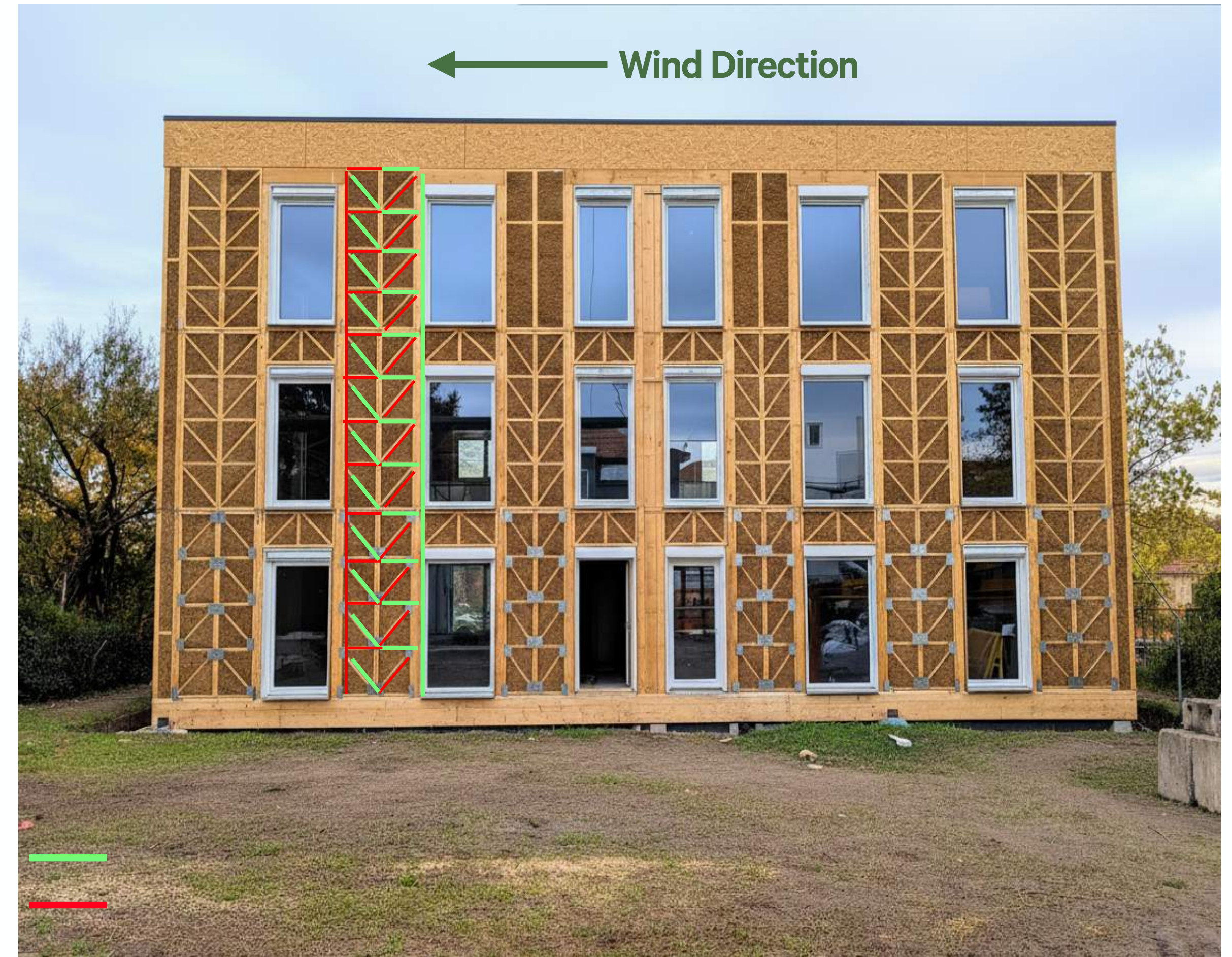
Existing building with a well-arranged EcoCocon wall bracing system: studs are aligned throughout all storeys, and the bracing is symmetric.
