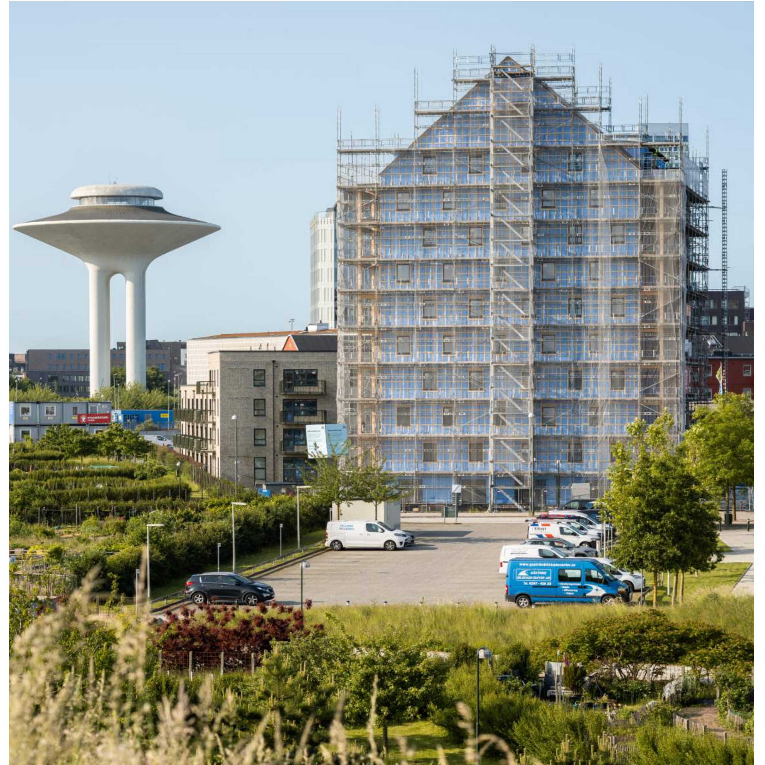
A 12-storey residential building in Malmö. Glulam and CLT superstructure is combined with EcoCocon external walls.
