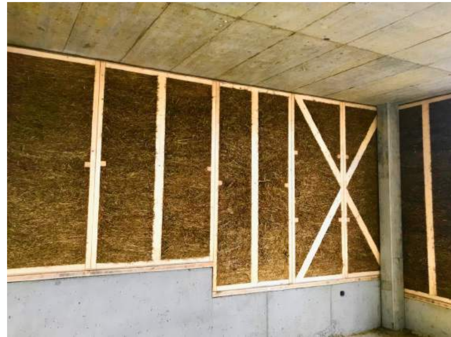
EcoCocon infill panels between concrete frame.
