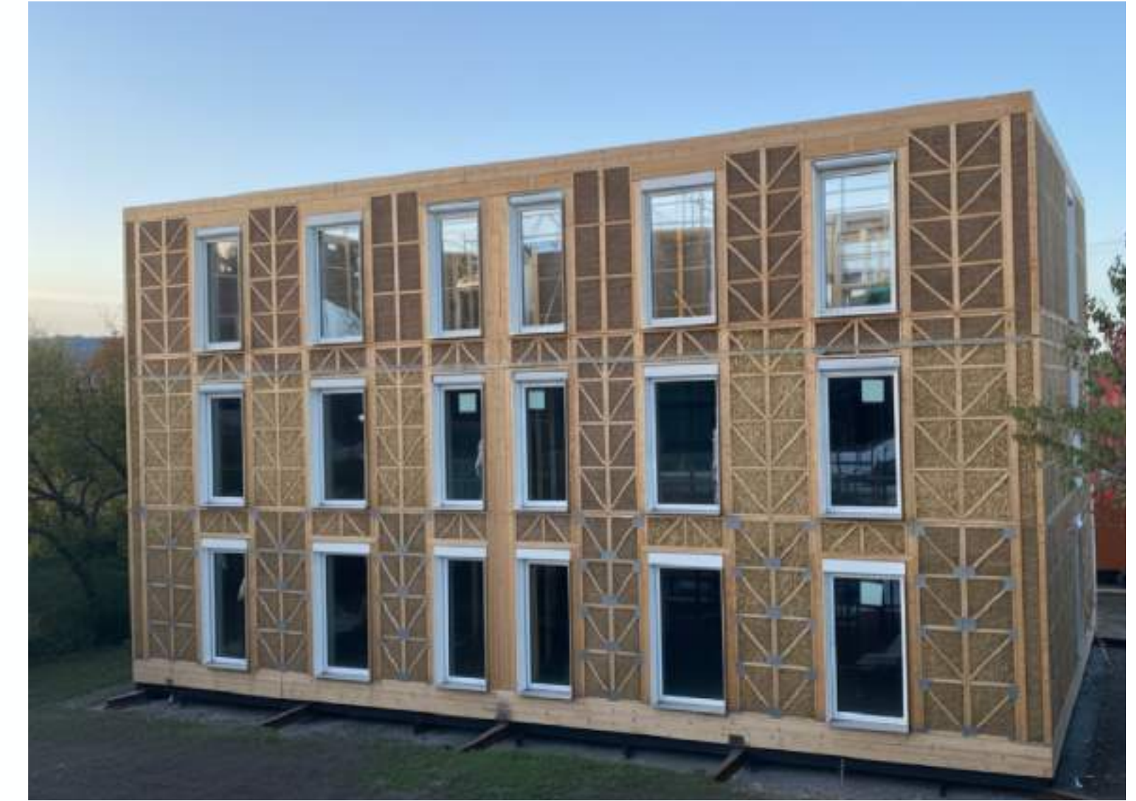
Loadbearing panel structure.
