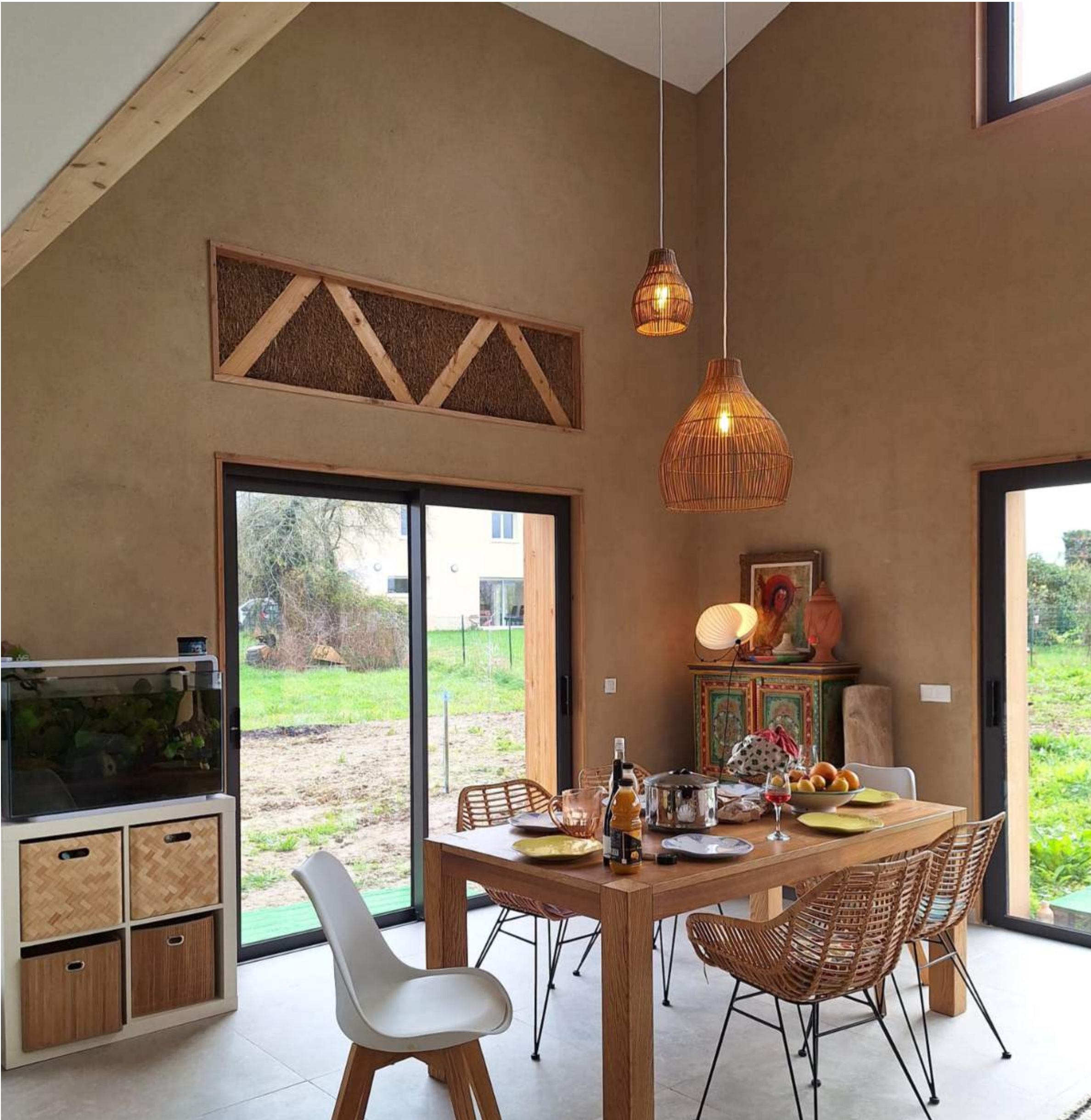
EcoCocon walls with clay plaster as the interior finish.
