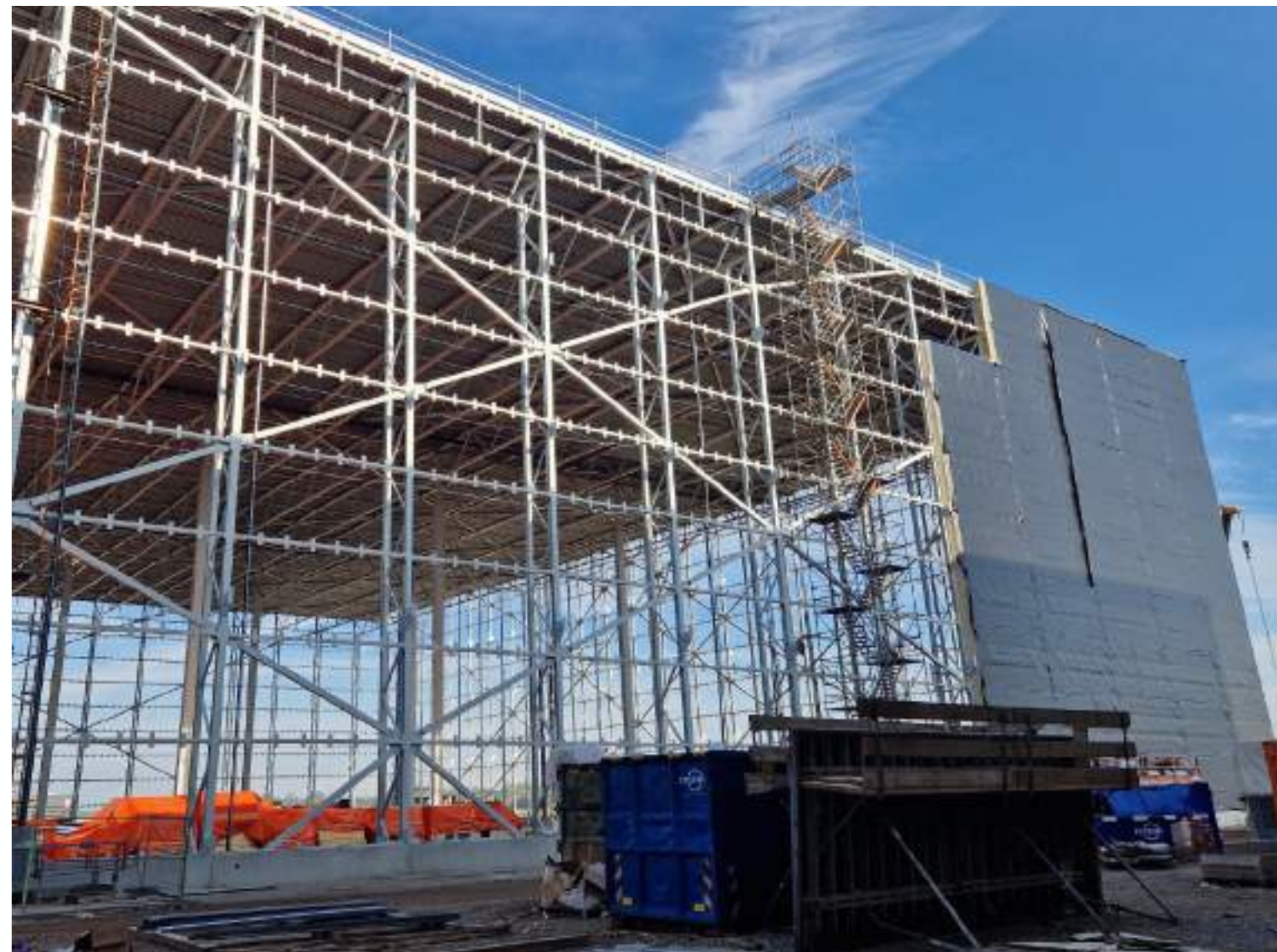
Self-supporting façade walls (external insulation façade).
