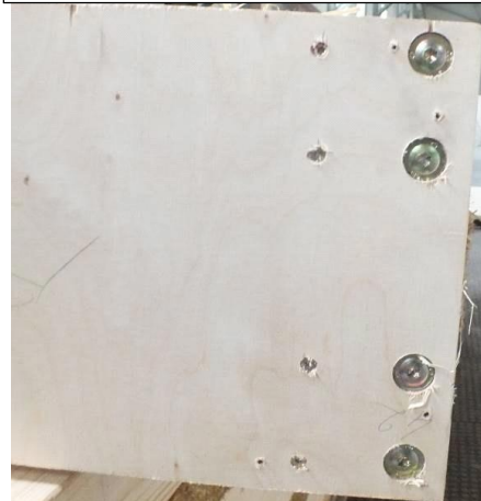
View of fixing of plywood to frame construction
