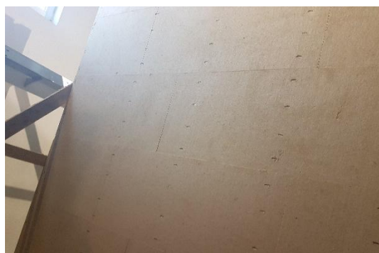
Covering of the wall by wood fibre boards
