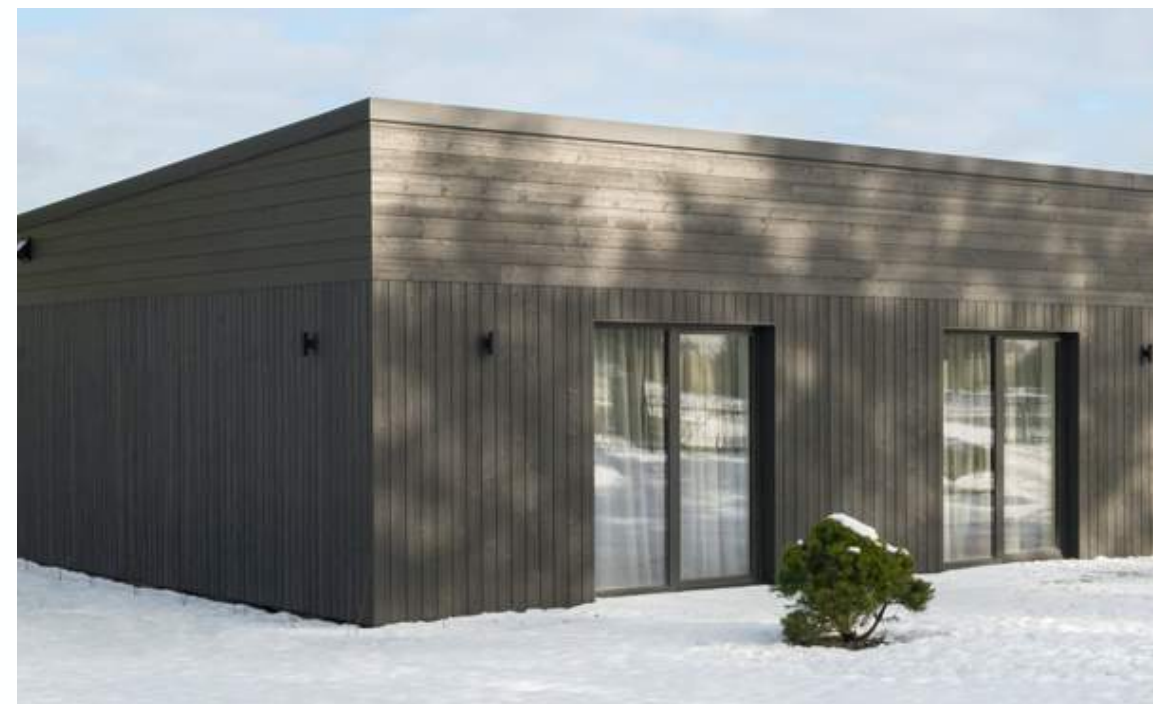
Ventilated wood cladding without gaps
