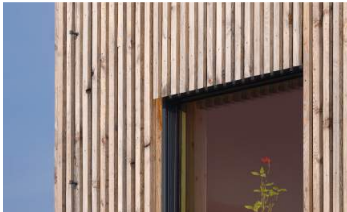
Ventilated wood cladding with gaps
