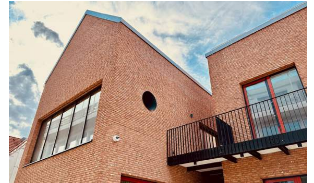
Ventilated brick facade
