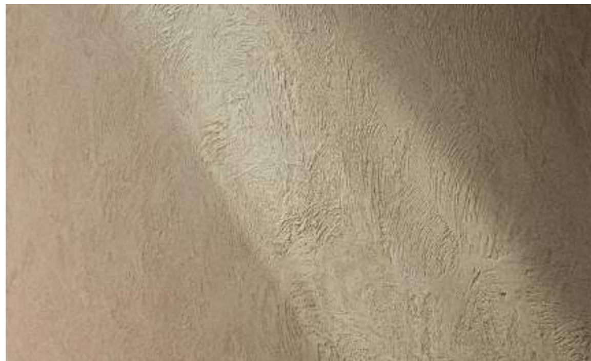
Decorative clay plaster
